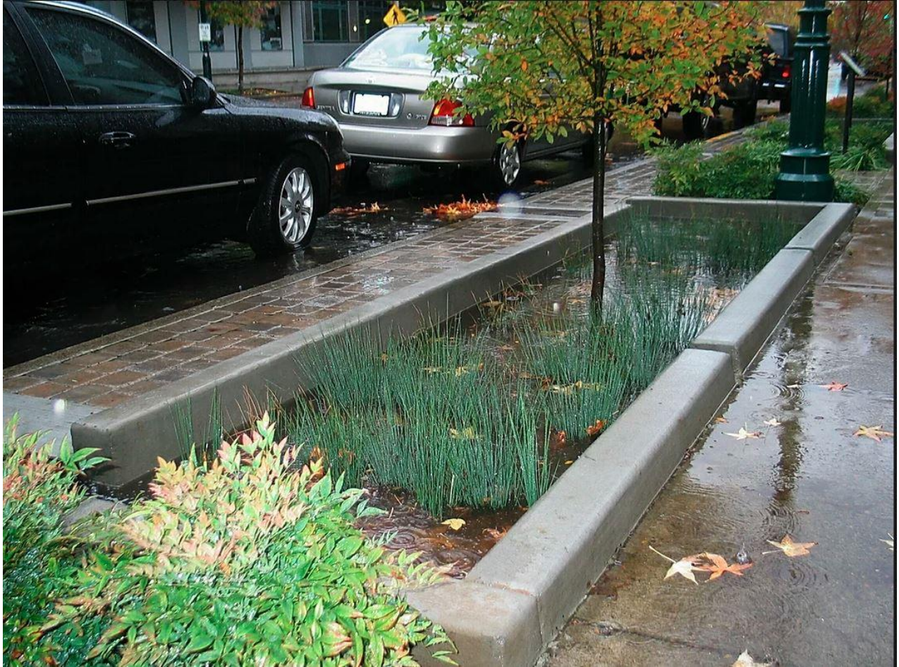
Figure 4: SW 12th Avenue Green Street during a rain event - Urbanraindesign.com
